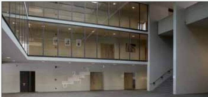
Smoke-proof glazed walls
